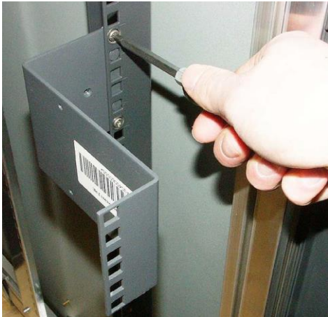
Figure 4: Installing the support bracket
