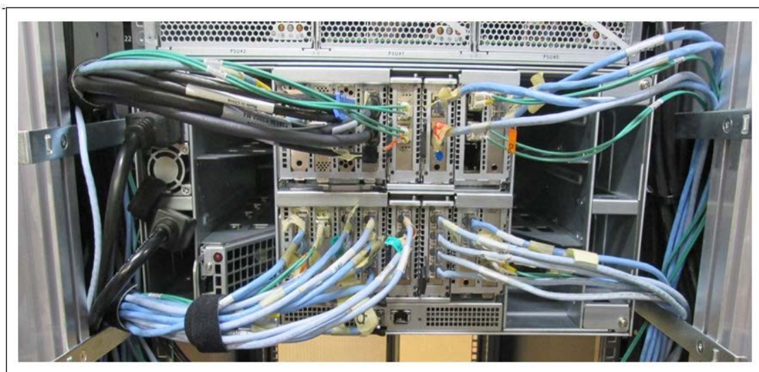
Figure G.2 Cable routing (recommendation)
