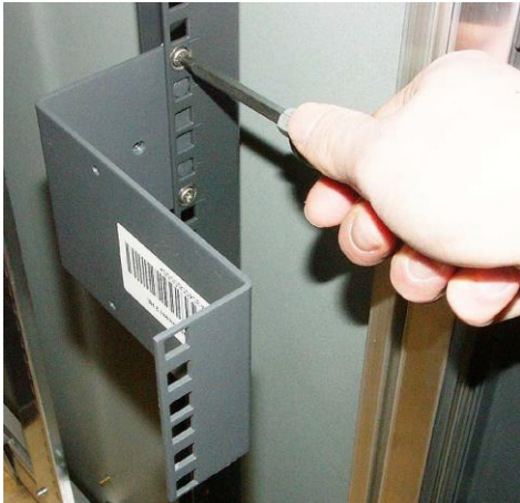
Figure 4: Installing the support bracket
