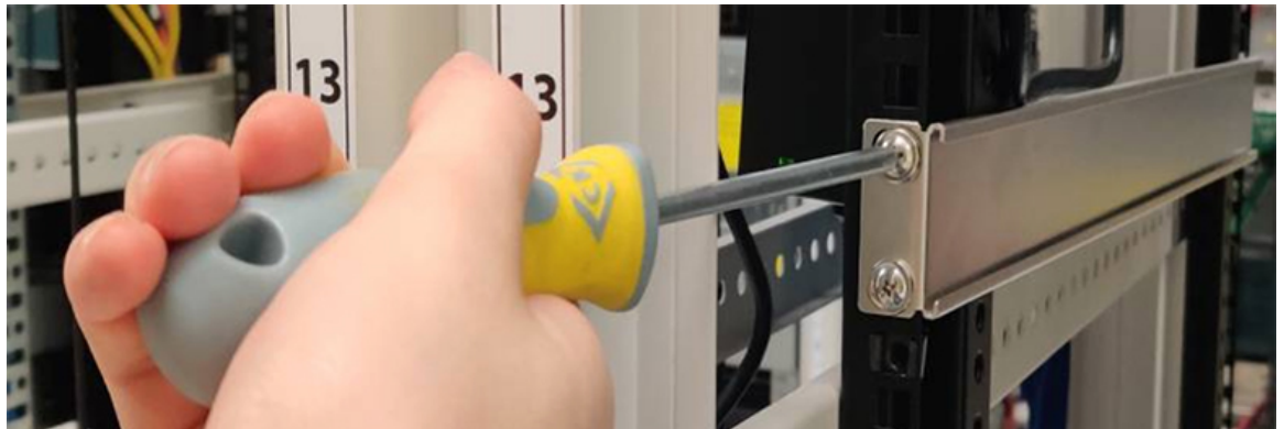
Figure 8: Attaching the left hand side rail.
