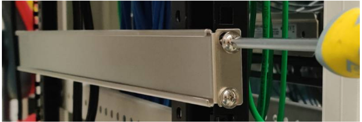
Figure 8: Attaching the left hand side rail.
